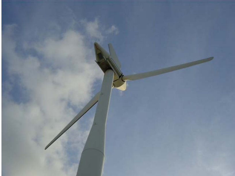
Photo 2. Wind turbine. Currently, an average wind speed of 9 mph for small wind generators (up to 100 kW in generating capacity) and 13 mph for large generators (measured at 100 ft above the ground) is considered necessary for the economical use of wind power. Photo by A.J. Both, New Jersey Agricultural Experiment Station.
