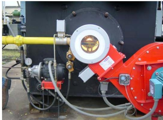
**Photo 4. Dual fuel boiler at Kube Pak, Allentown, NJ.**
